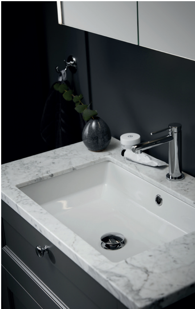
The basin is recessed in the stone work top which gives a 10 mm thin stone edge on the inside even though the stone worktops are 30 mm.
